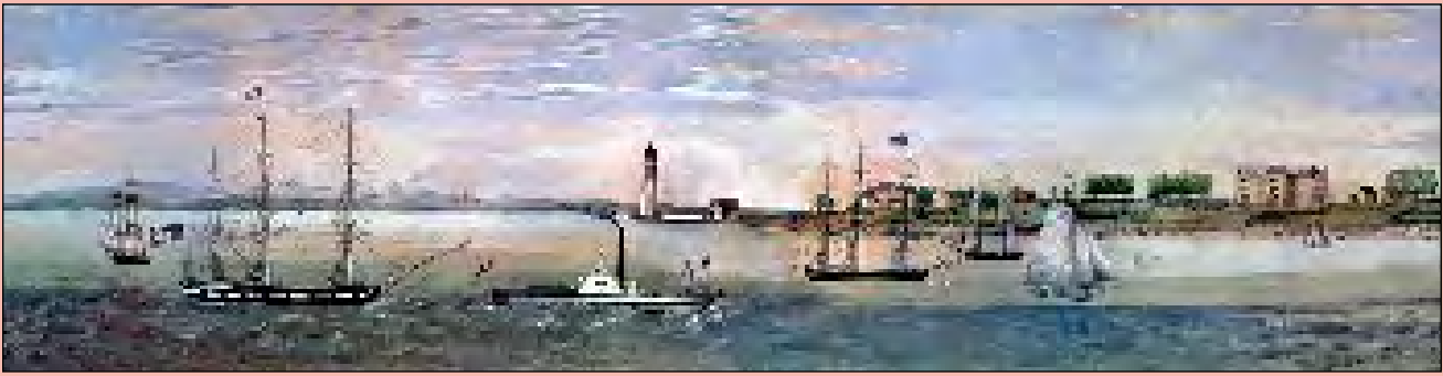
Leaving the harbor, 1845. At the southern tip of New Bedford's peninsula, extending into Buzzards Bay, is the Clark's Point lighthouse (center). The prominent building at far right, surrounded by tree groves, is the city's alms house or "Poor Farm." Under sail is an inbound coaster, and next, the whaleship Janus. In the foreground, the whaleship Niger returns from a voyage under tow of the steamer Massachusetts; and a pilot boat brings up the rear. — Russell & Purrington panorama. New Bedford Whaling Museum.
